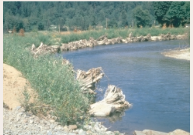
Figure 8.47: Completed system after one year. Note dramatic willow growth from vegetated geogrid.
